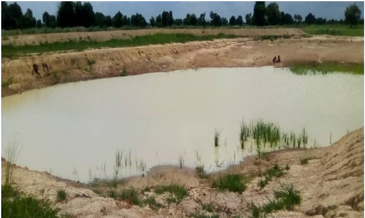
Figure 2.2: Small Earth Dam at Katigri
