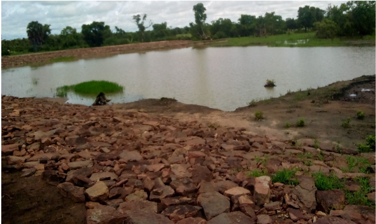
Figure 2.1: Small Earth Dam at Dabozesi
